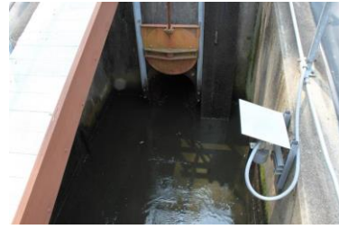
Exhibit 4-4. Flow Sensor and Discharge Valve
