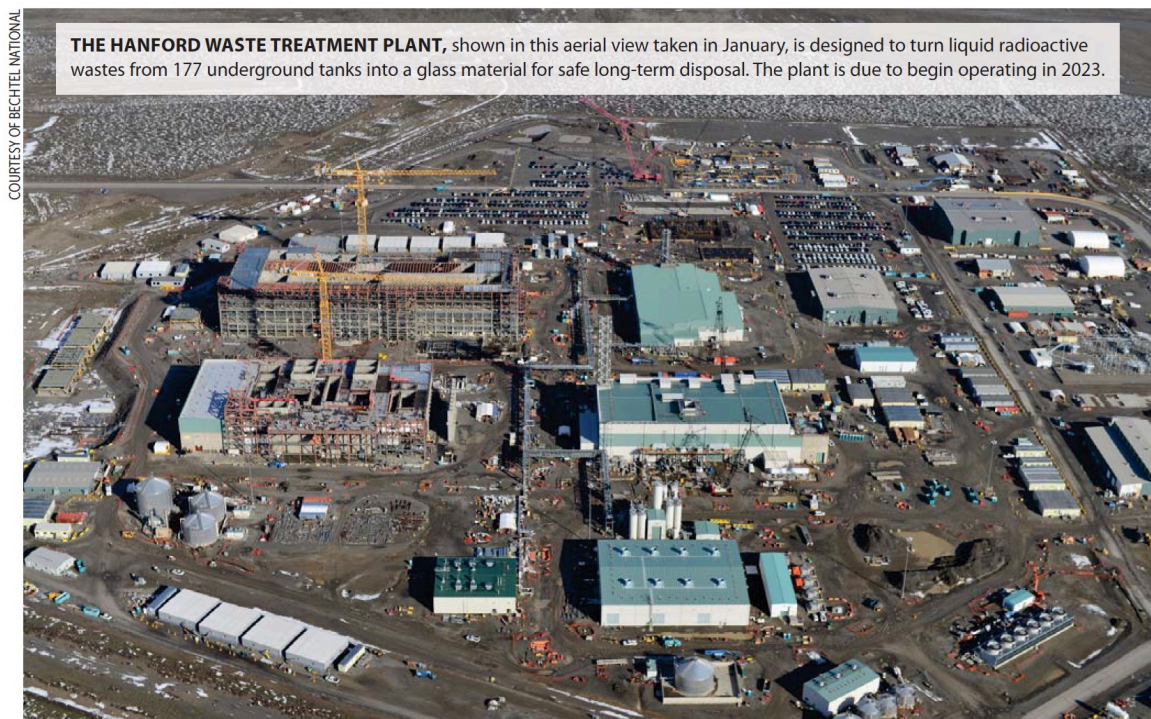
Fig. 1.3 - the Hanford waste treatment plant in January 2017 [6]
