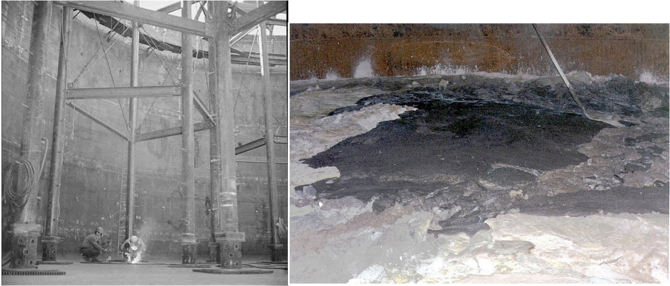
Fig. 1.2 Hanford waste tank construction (left) and present interior surface of a waste tank (1989)
