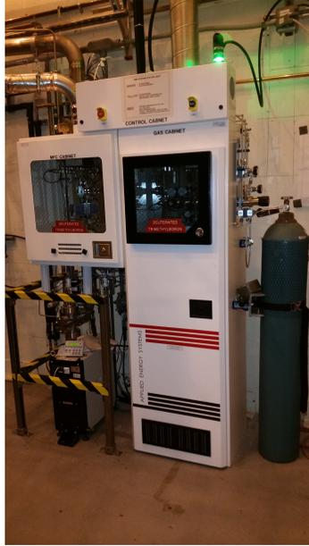
Fig. 1. dTMB gas management layout for the boronization of NSTX-U
