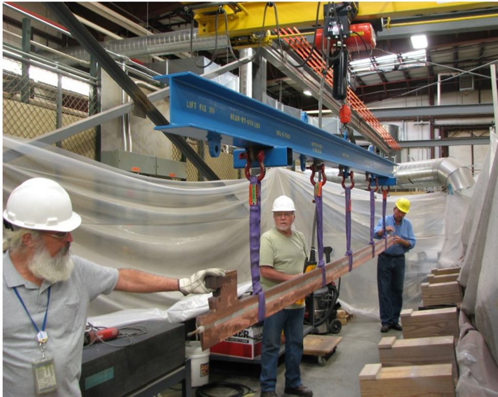
Figure 31 Completed Conductor Loaded Into Transport Crate
