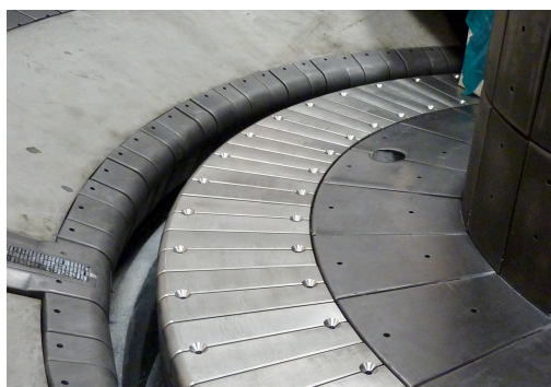
Fig. 5 Photograph showing row of TZM PFC tiles on inboard lower divertor in NSTX. Gap for CHI can be seen to the left of the tiles.
