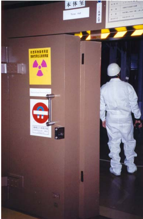
Figure 5. A radiation shielding door at entry to the JT-60 torus hall.
