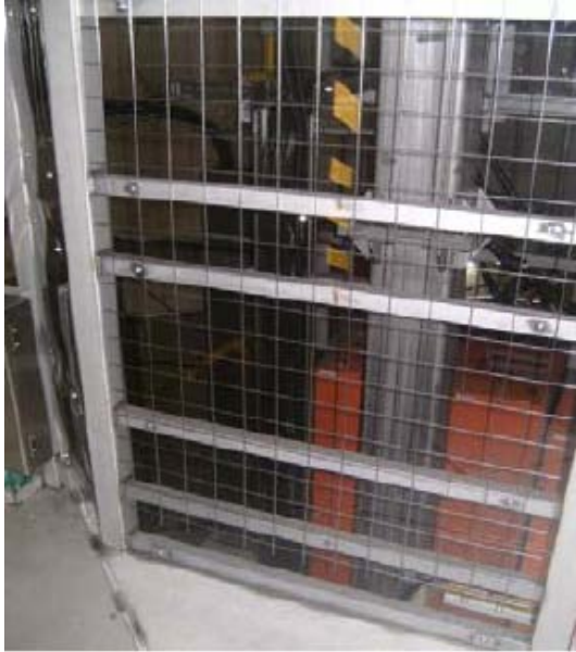
Figure 2. Protective panels on walkways near the LHD machine.
