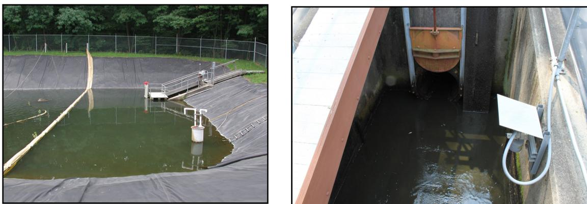
**Exhibit 4-3. PPPL Retention Basin; Flow Sensor, Discharge Gate**
