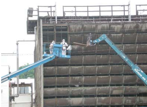
Exhibit 3-23 Worker Using Bucket with Safety Equipment for Cooling Tower Demolition Project
