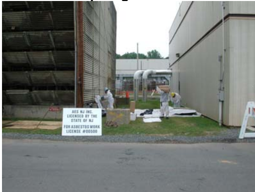
Exhibit 3-22. Workers Preparing Asbestos-Work Site
