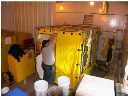
Exhibit 6-9. An Enclosure in HAZMAT Building for Lead Separation from Concrete Shielding Blocks
