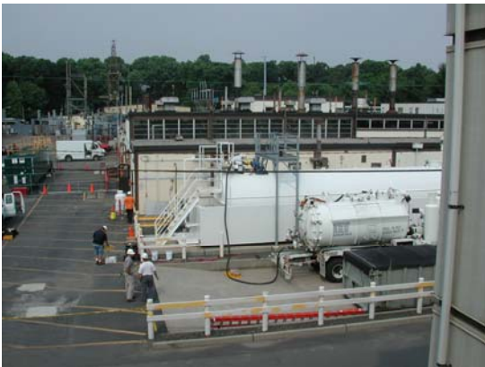
Exhibit 3-18 Cleaning AST-1 Looking West Toward Boiler Room
