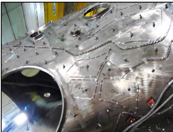
Figure 2. Installation of magnetic flux loops on a NCSX vacuum vessel segment.
