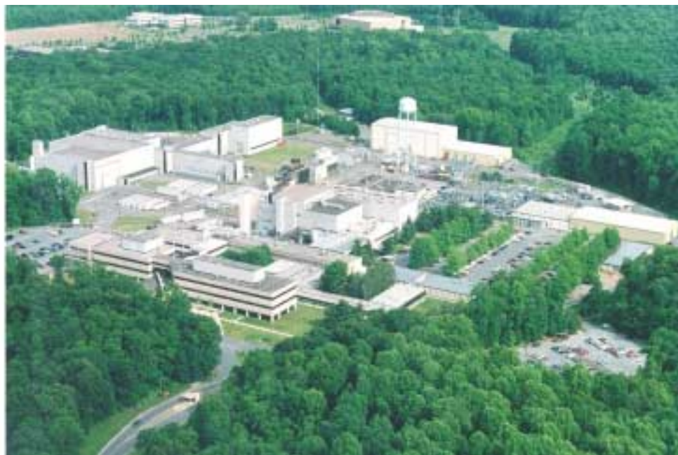
Exhibit 2-3. Aerial View of PPPL
