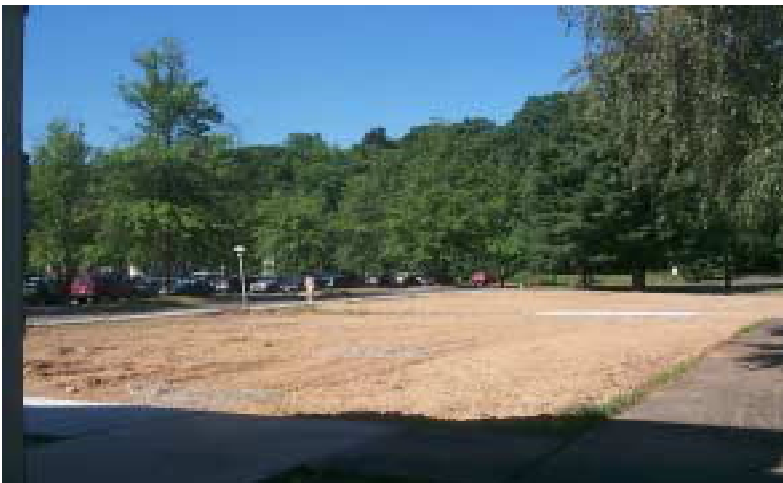
Exhibit 3-4. Demolition of MOD I —materials for recycling and landfilling
