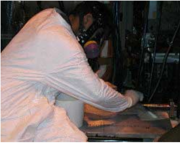
Fig. 2 Application of strippable paint to a lead oxide contaminated surface.
