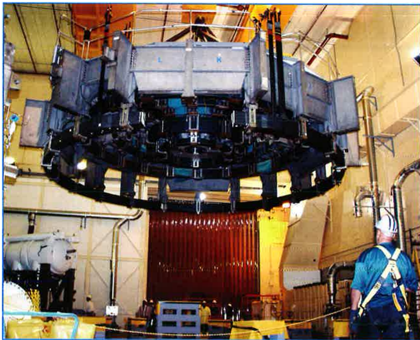
The disassembly of the Tokamak Fusion Test Reactor (TFTR) at PPPL progressed. On November 8, the umbrella structure and upper magnetic poloidal-field coils were lifted off the top of TFTR. Workers used the 110-ton capacity overhead bridge crane to make this 92-ton lift. The structure and coils were removed as part of the machine's disassembly, which is expected to be completed by September, 2002.
