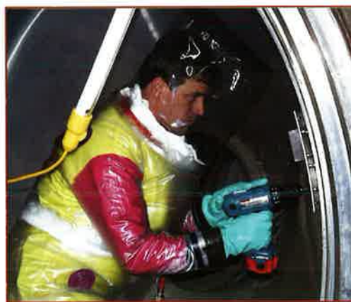
Figure 14. A technician practicing in the TFTR vacuum vessel mock-up in preparation for entry into the contaminated TFTR vacuum vessel.
