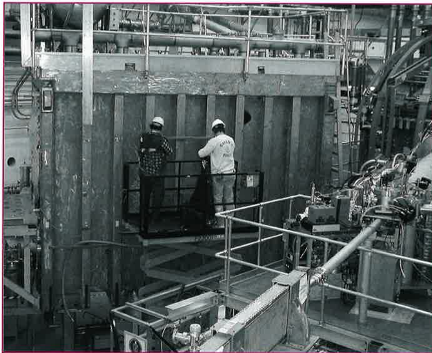
Figure 5. NSTX beamline undergoing modifications and installation.
