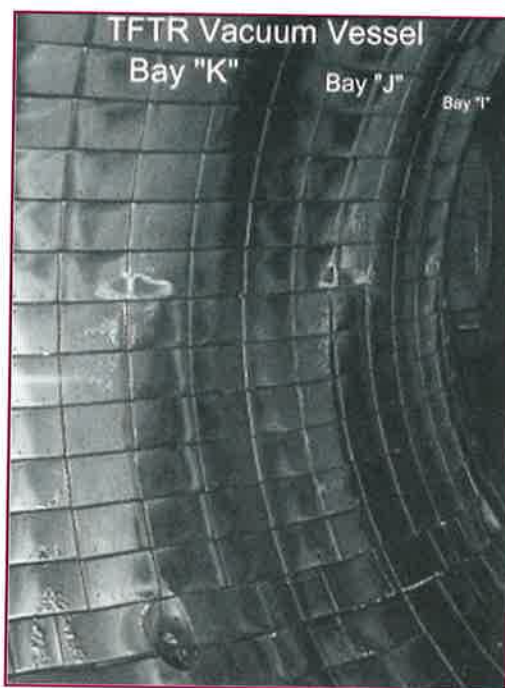
Figure 11. Tiles making up the bumper limiter on the inside wall of TFTR showing flaking developing at bay "K" in the lower left corner.
