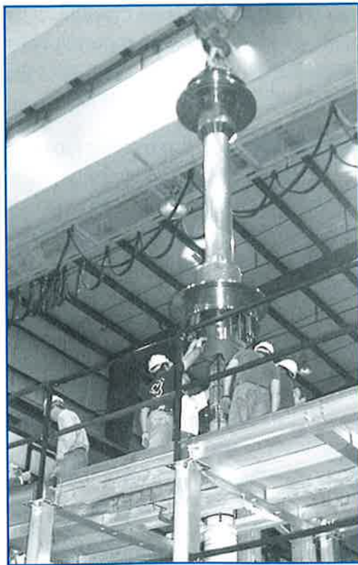
Figure 3. Completed NSTX center stack.
