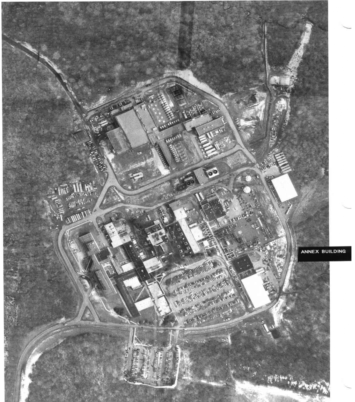
FIGURE 13. 1975 AERIAL OF PPPL INCLUDING ANNEX BUILDING
