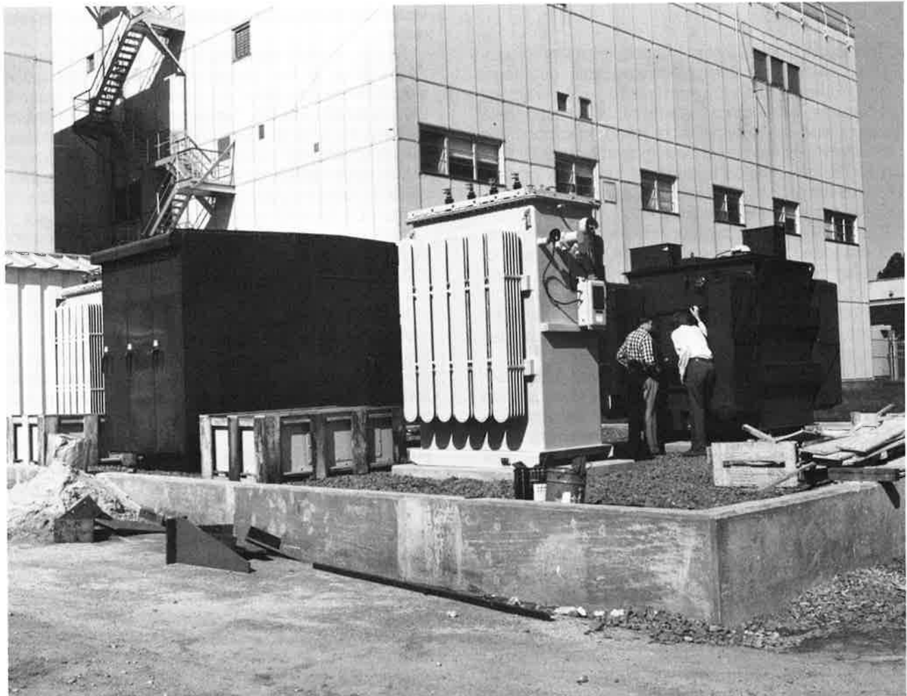
Figure 33. PLT 55-MHz ICRH high-voltage power supply under construction.
