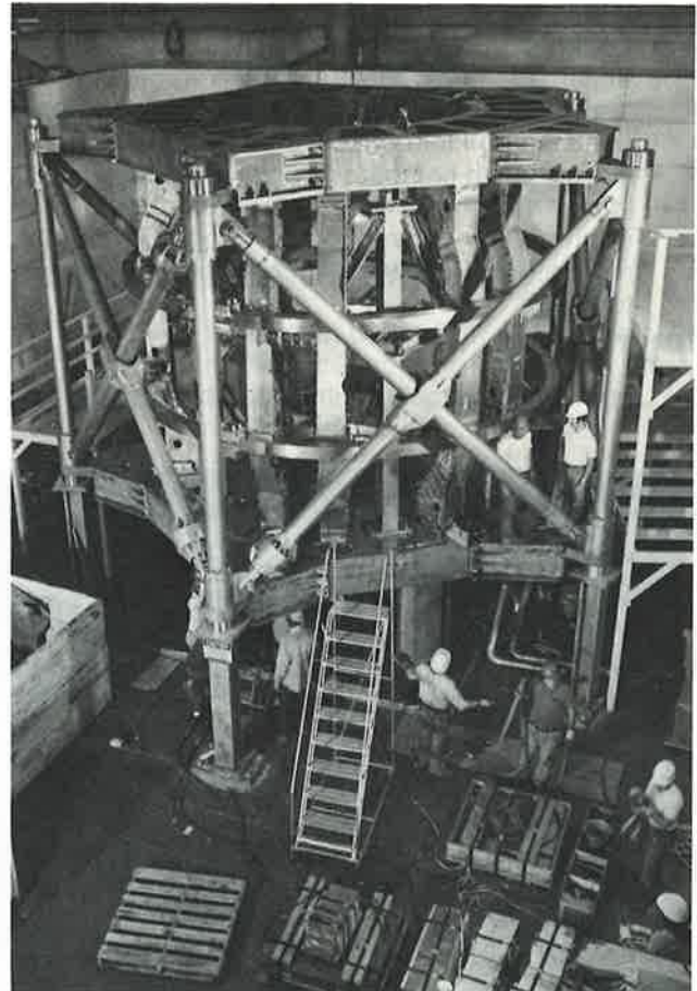
Figure 51. Preassembly of PDX outer structure and TF coil cases.
