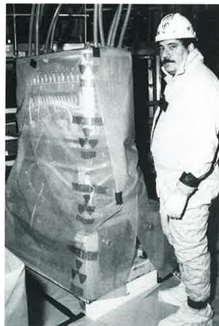
Reworking of the neutral-beam ion sources was performed safely within a temporary work area set up in the TFTR Test Cell.
