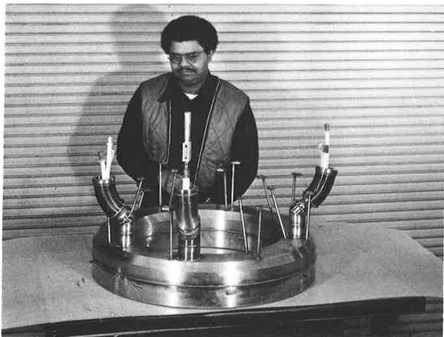
754001 Fig. 8. New 260,000 ampere - turn FM-1 divertor field coil.
