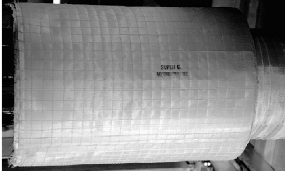
Figure 9 – Microtherm Blanket Covering OH and PF1a Coils
