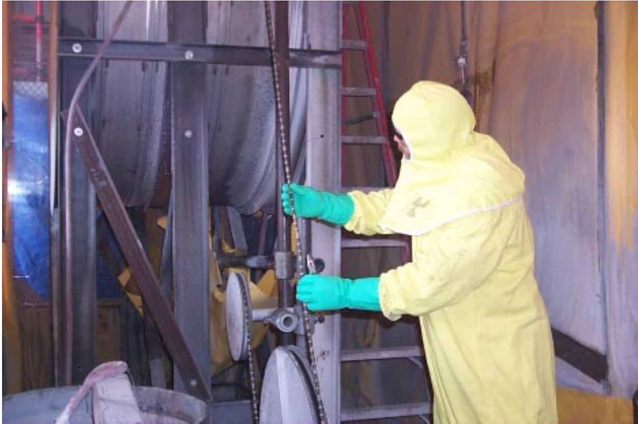
Figure 4 - Diamond Wire Rope and Pulleys
