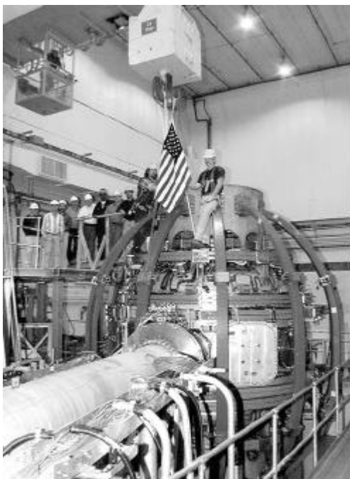
Figure 1. NSTX During Construction in January, 1999
