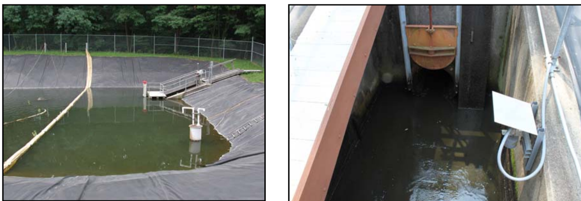
Exhibit 4-3. PPPL Retention Basin, Flow Sensor, Discharge Gate
