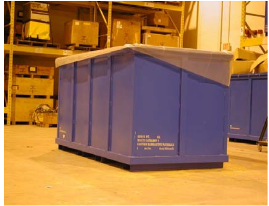
Exhibit 5-5. B-box with Liner in RWHF for Shipping Radioactive Waste to Clive
