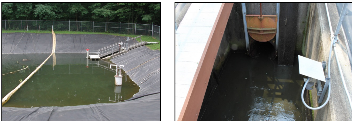
Exhibit 4-3. PPPL Lined Surface Impoundment/Basin, Flow Sensor, and Discharge Gate
