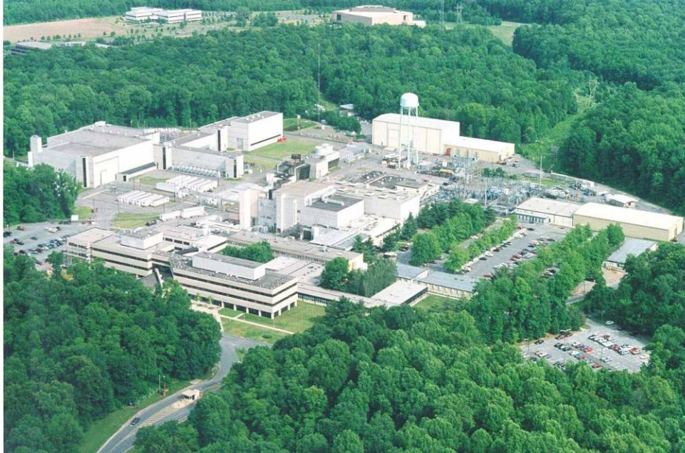
Exhibit 1-3. Aerial View of PPPL
